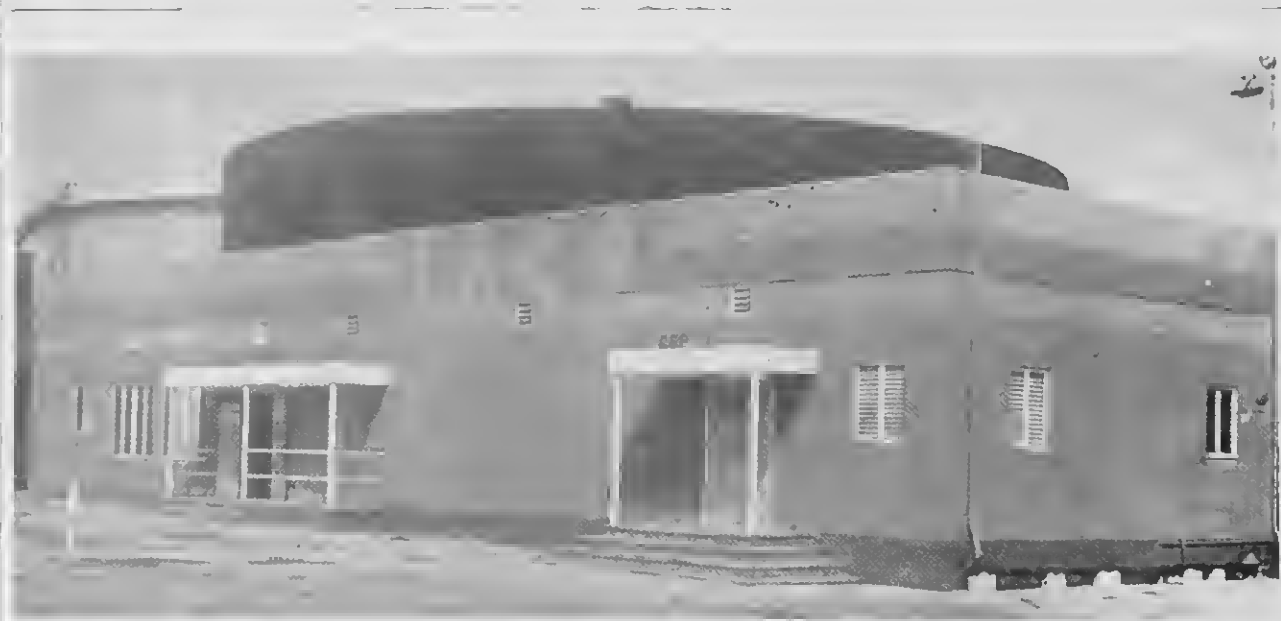
START AND FINISH POINT: Pictured is the new Reception Center which will be the starting and finishing points of the family tour program. Tour guests will gather at the Center for an introductory talk and upon completion of their tour through the refinery will be served refreshments here.
